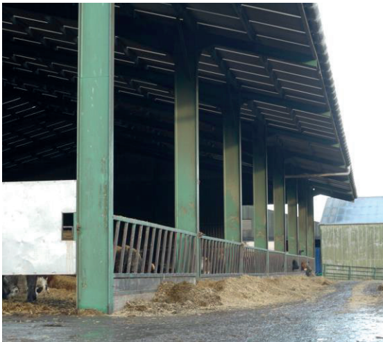
External feed barrier with overhanging roof
